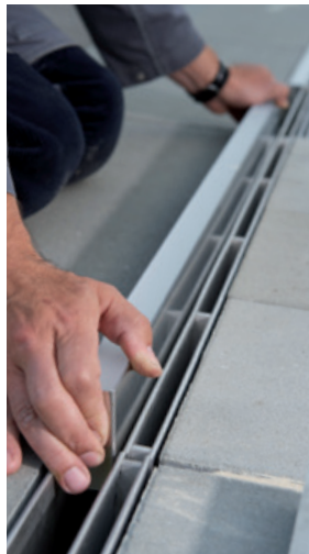
Mounting the LED elements in the slotted frame
