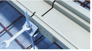
The channel is tightened with nuts (M10) at the point of contact to secure it against displacement and protrusion. This requires special care to align the channel line and transitions. The channel line should not be loaded or moved until the concrete has cured.
